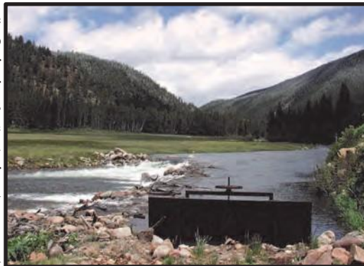
Diversion Structure on Crystal Creek
