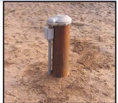
Standard domestic water well in Weld County
